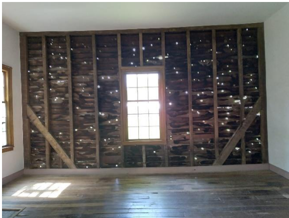
Inside the Carter House farm office building.
